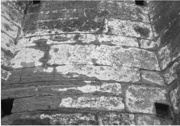
Fig. 14.3 Dirina massiliensis forma soreciata on calcareous church wall to show extensive development of calcium oxalate at the thallus-substrate interface. (Photograph by M. R. D. Seaward.)
